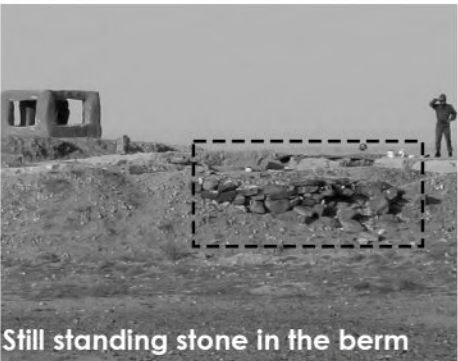
Sand and stone berm wall
