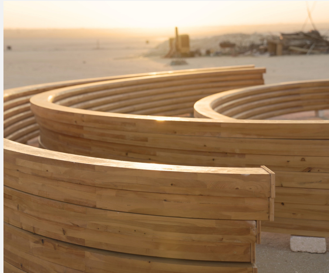
Wooden Ribs Detail
