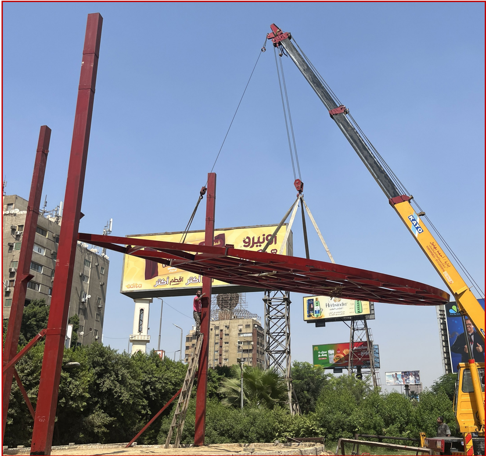
INSTALLING THE FRAME
