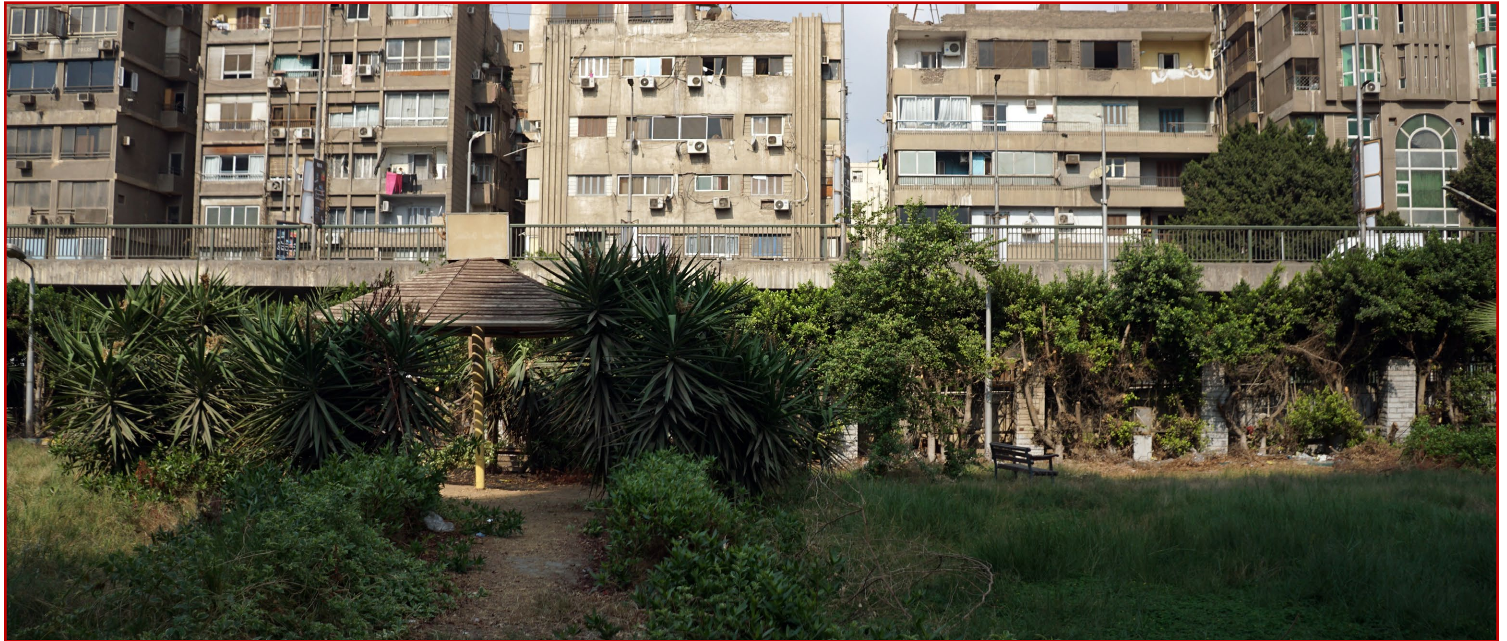
EXISTING SITE PRIOR TO CONSTRUCTION OF THE PERGOLA
