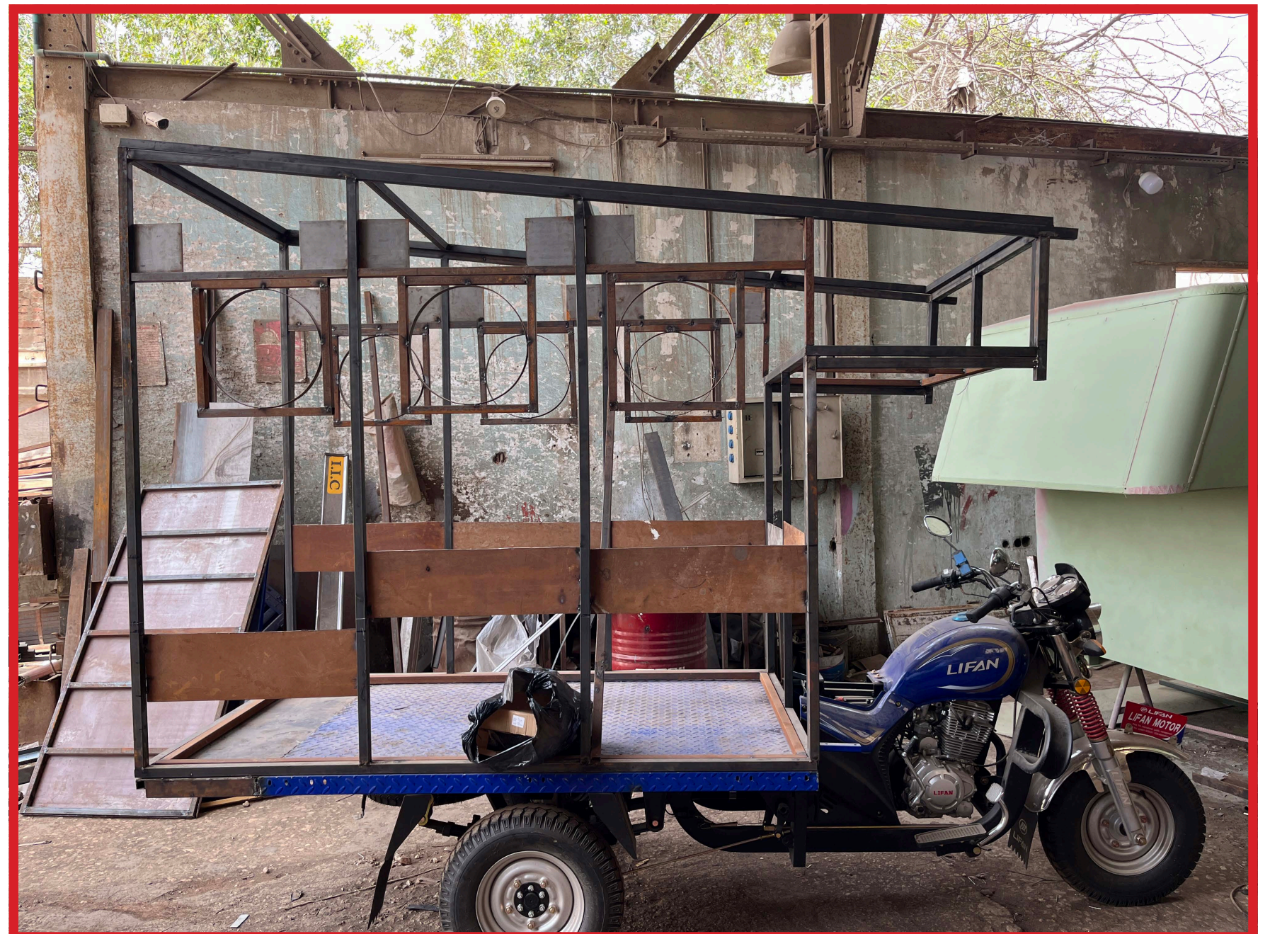
BUILDING OF THE METAL STRUCTURE ON TOP OF THE BASE
